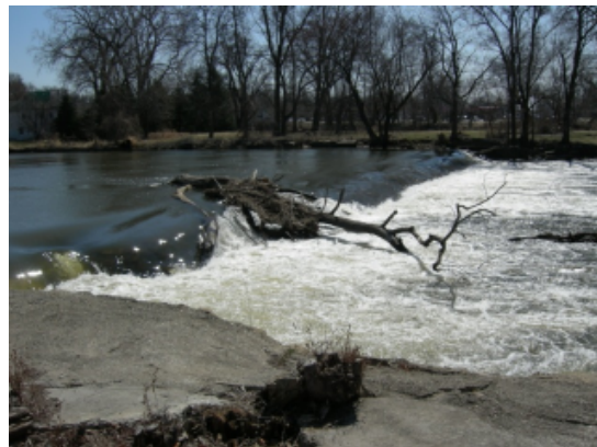
The Momence Dam on the Kankakee River.
